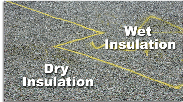
Control image, wet sections marked for removal
