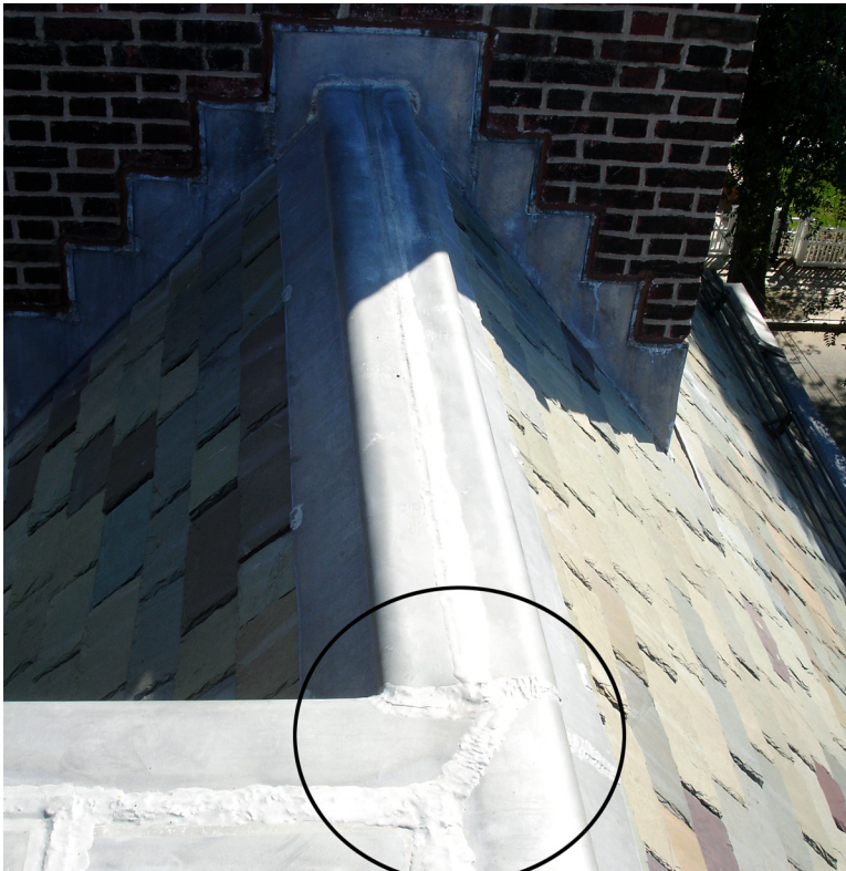
G16: cracked solder joint
