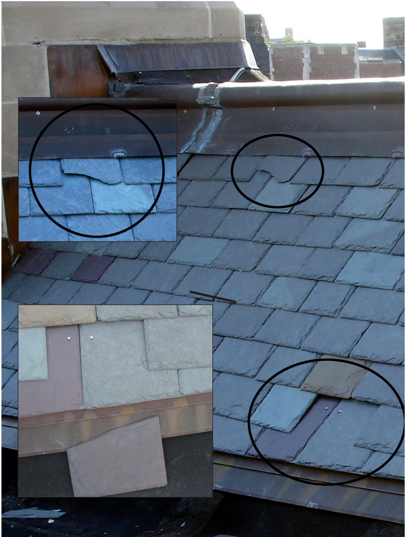
C5: broken slate, missing slate
