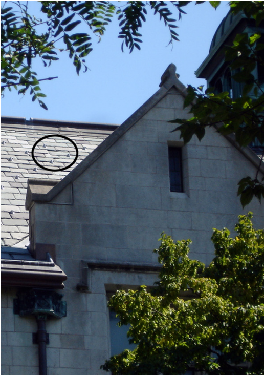
C1: cracked slate
