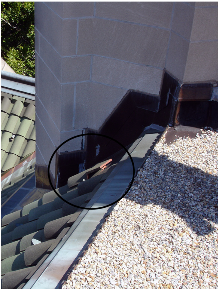
VS10: tile missing, nailer exposed
