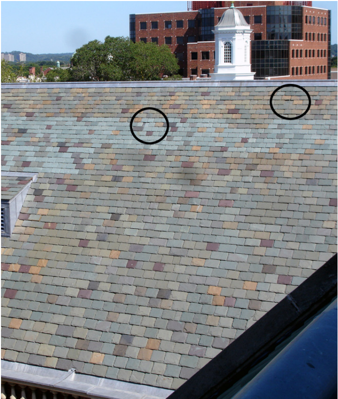
B6: slate missing four courses down from ridge and nine courses down from ridge
