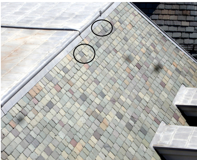
M4: slate slipping and broken
