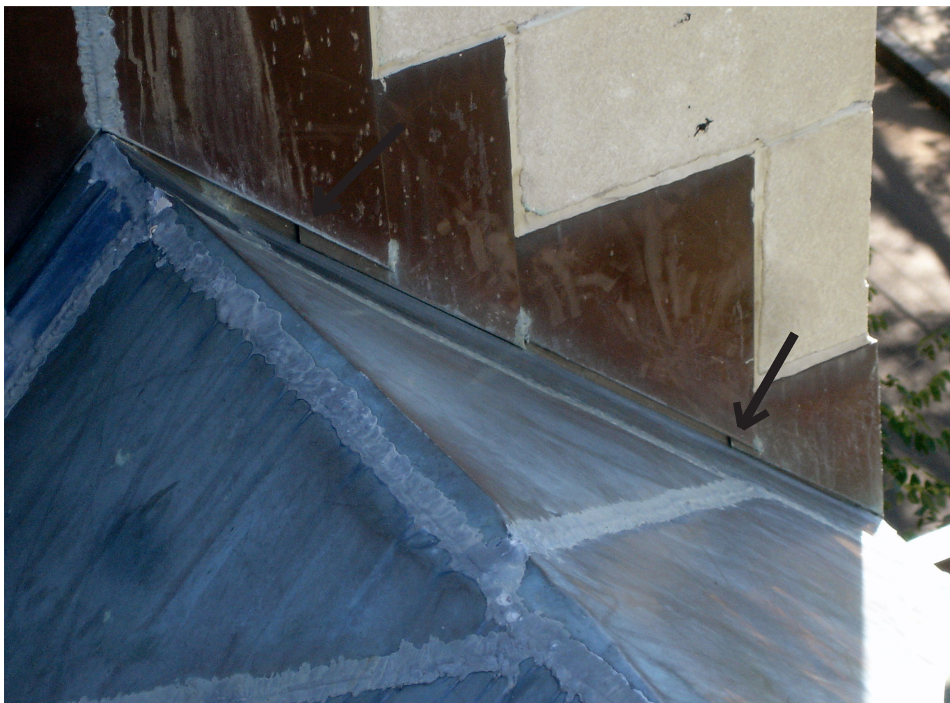
VS11: step flashing appears lapped against flow
