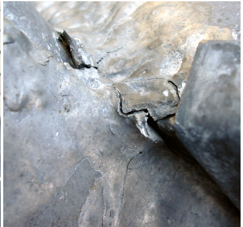
G2: close up of cracked solder
