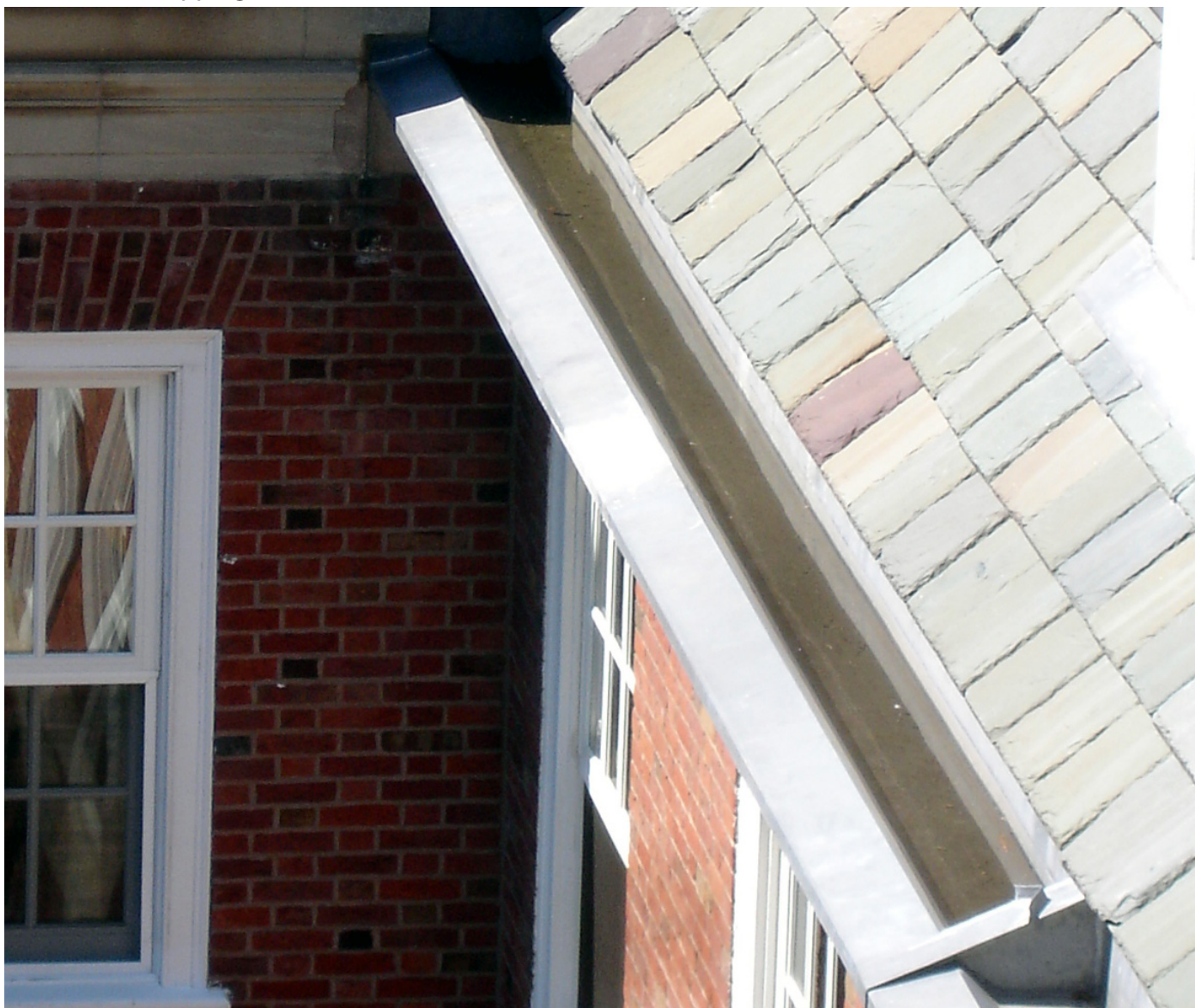
G10: blocked gutter
