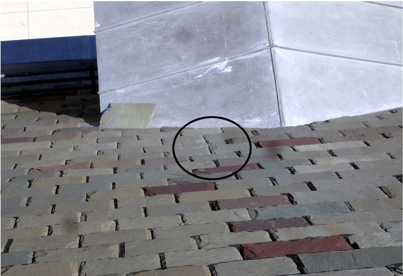
B2: 1 missing slate, slate resting on dormer roof
