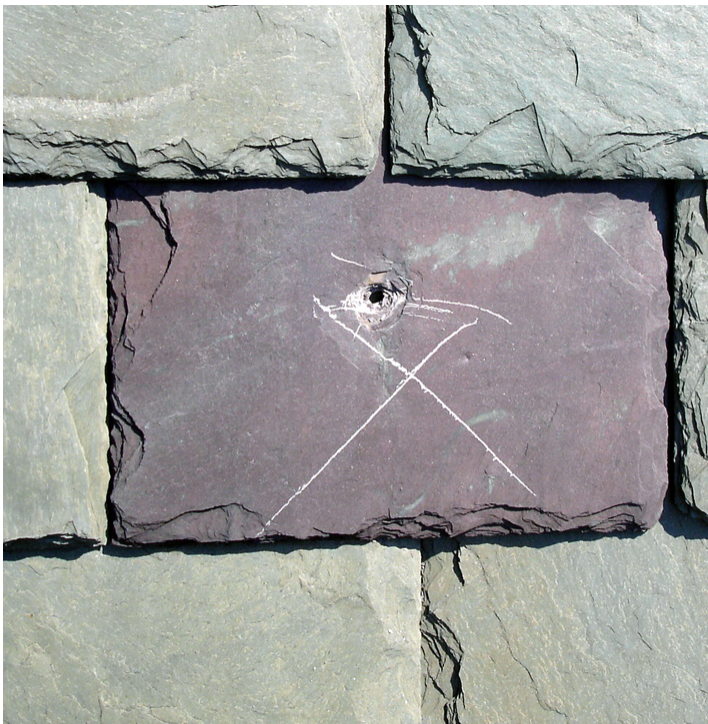
G4: exposed hole in one slate
