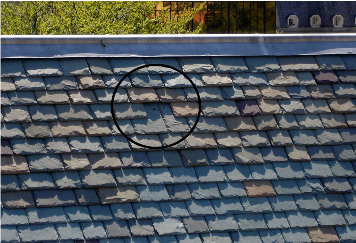
B6: close up, one slate missing four courses down from ridge
