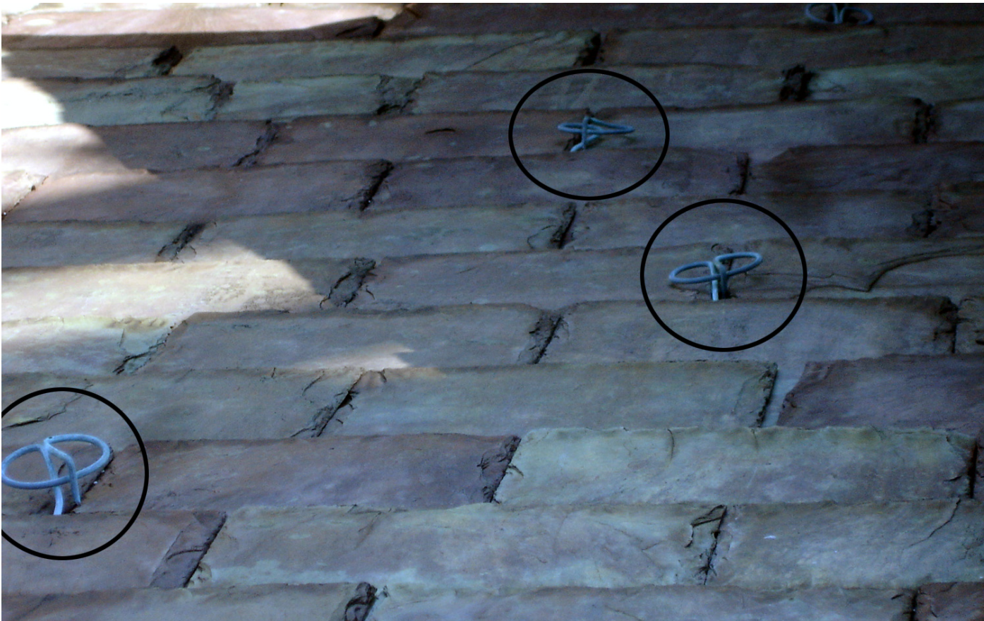
C3: flattened wire snow guards
