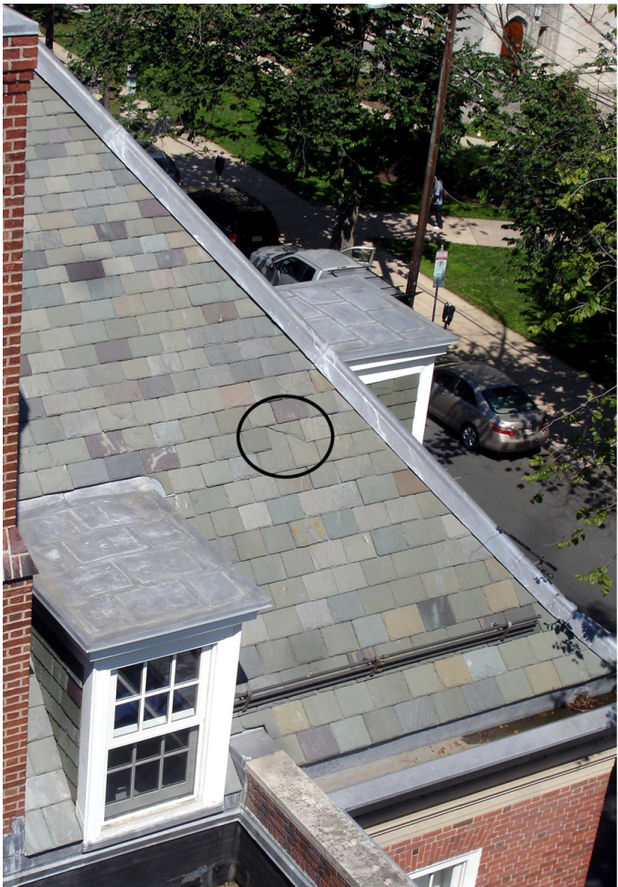
G1: one slate broken twelve courses up from gutter
