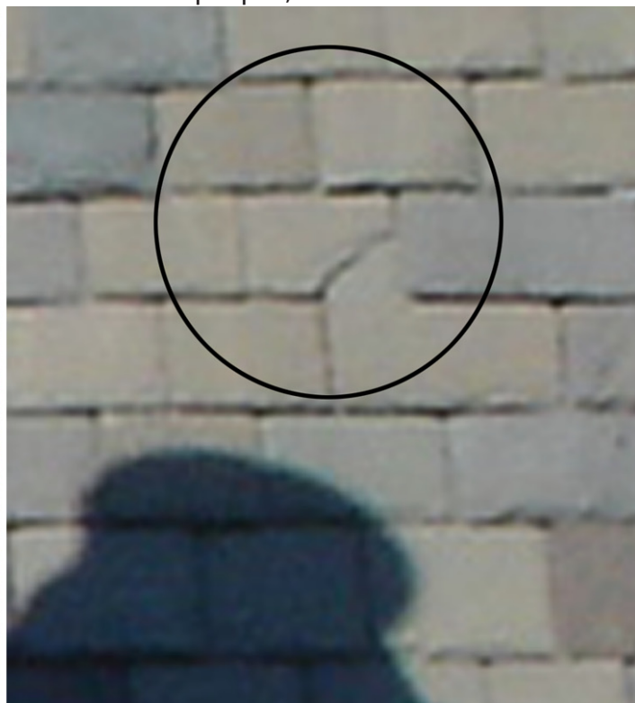
G12: metal strap repair, three observed on roof
