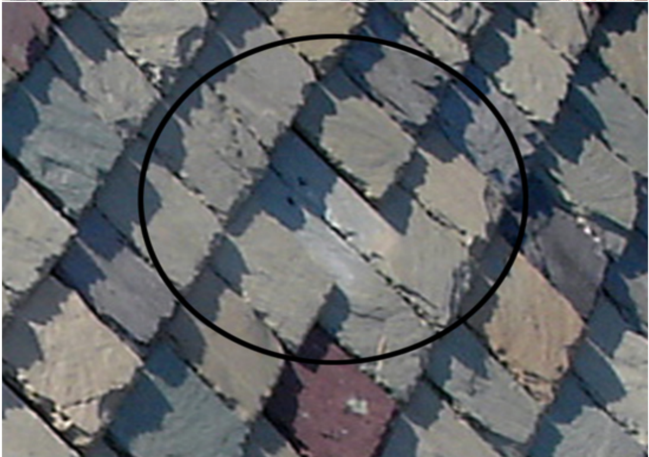
G8: one broken/ missing slate, slate resting on dormer roof
