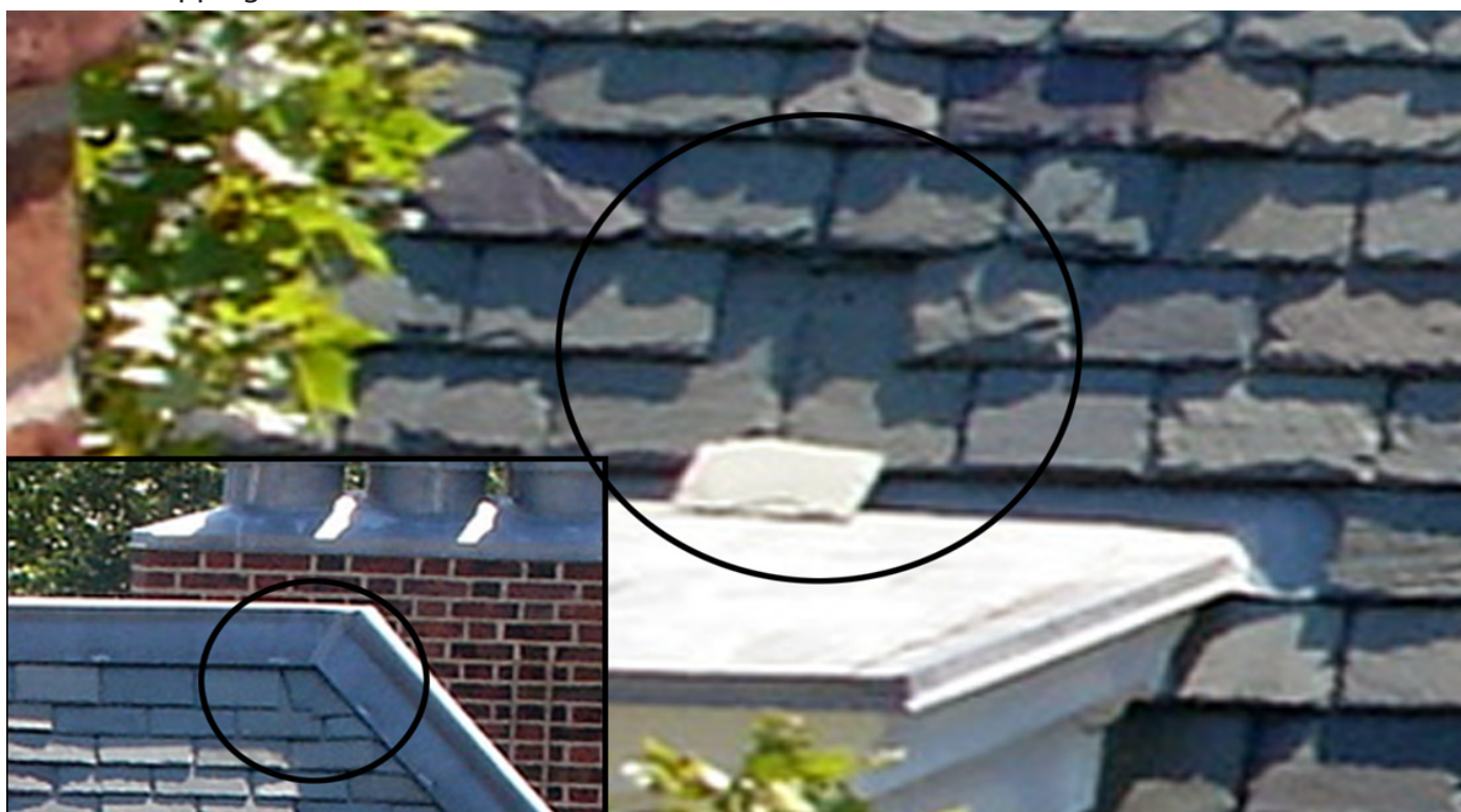
G13: slate has fallen out and is resting on dormer roof
