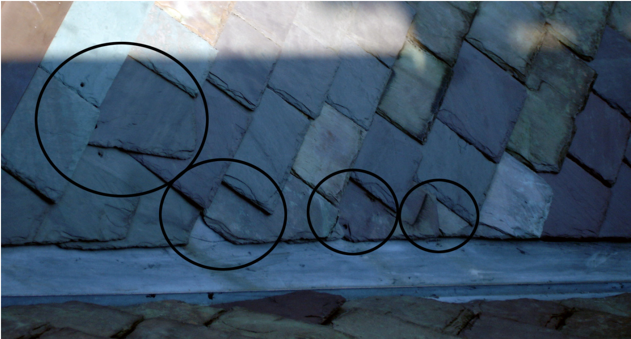
C7: broken and missing slate (portion of original slate roof)
