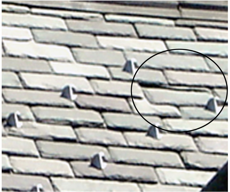
C1: close up of cracked slate
