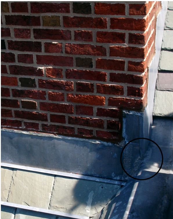
G2: cracked solder
