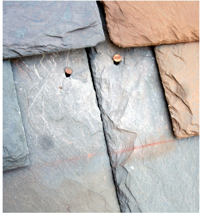
G5: missing slate two courses down from ridge
