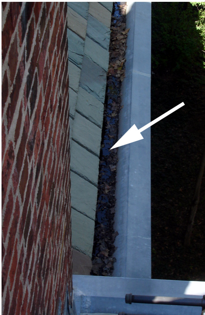
G11: debris blocking gutter outlet
