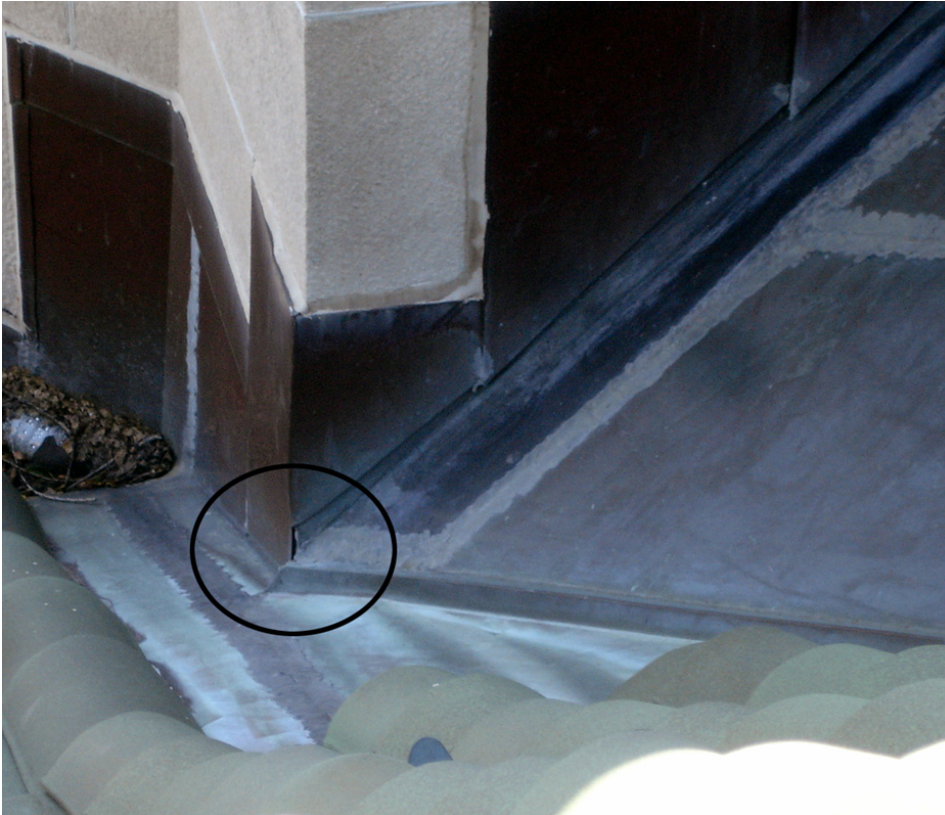
VS11: copper chimney flashing appears open at corner
