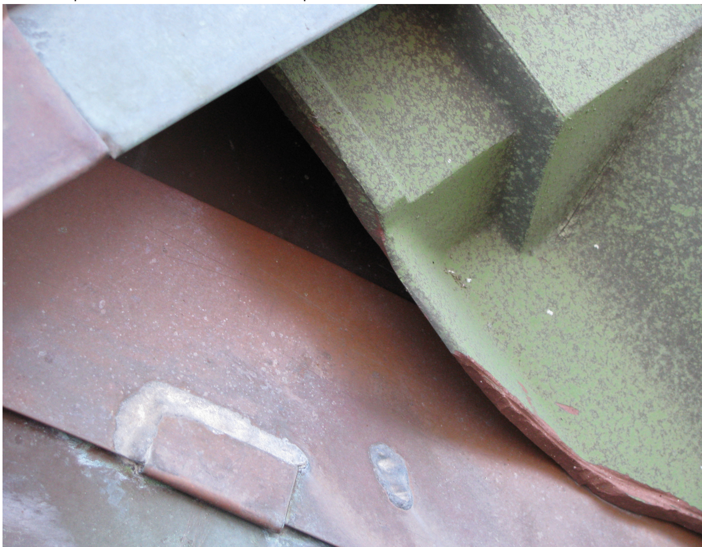
VS6: missing flat top tile piece
