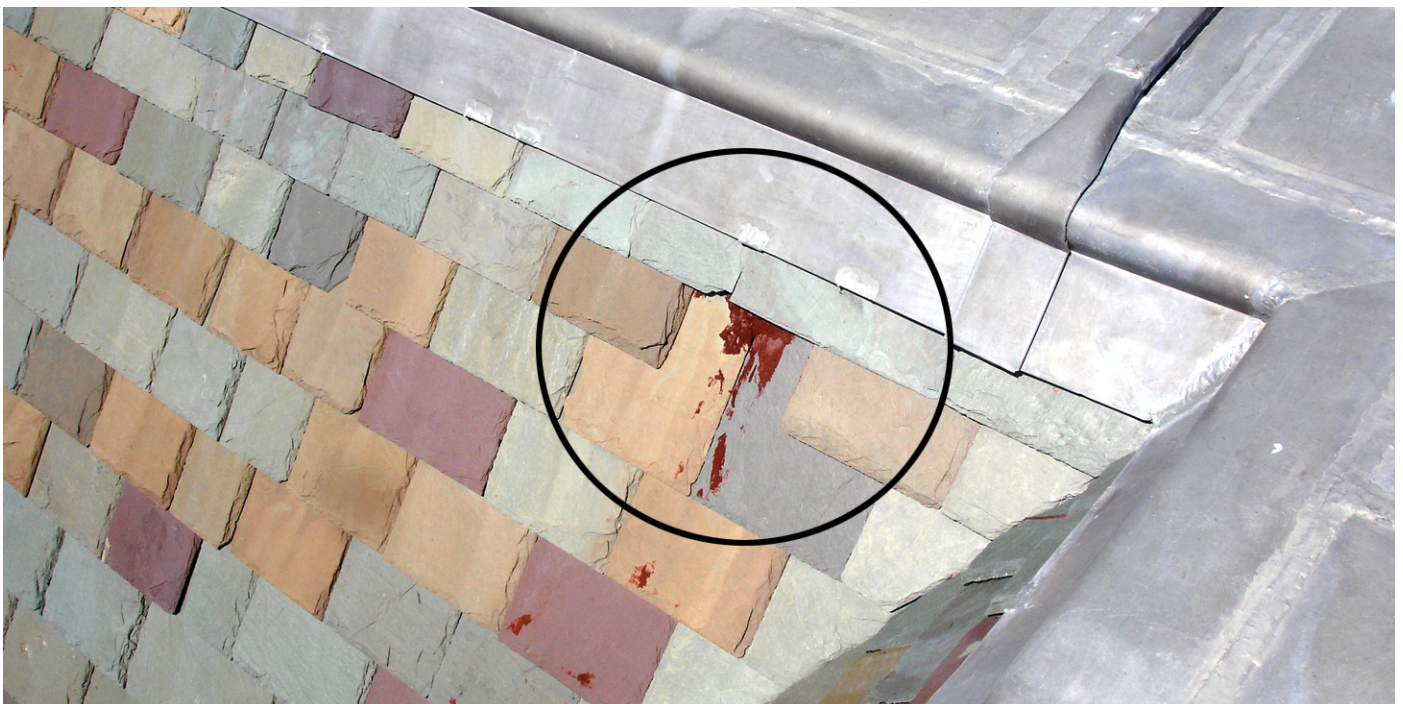
B4: 1 missing slate near ridge
