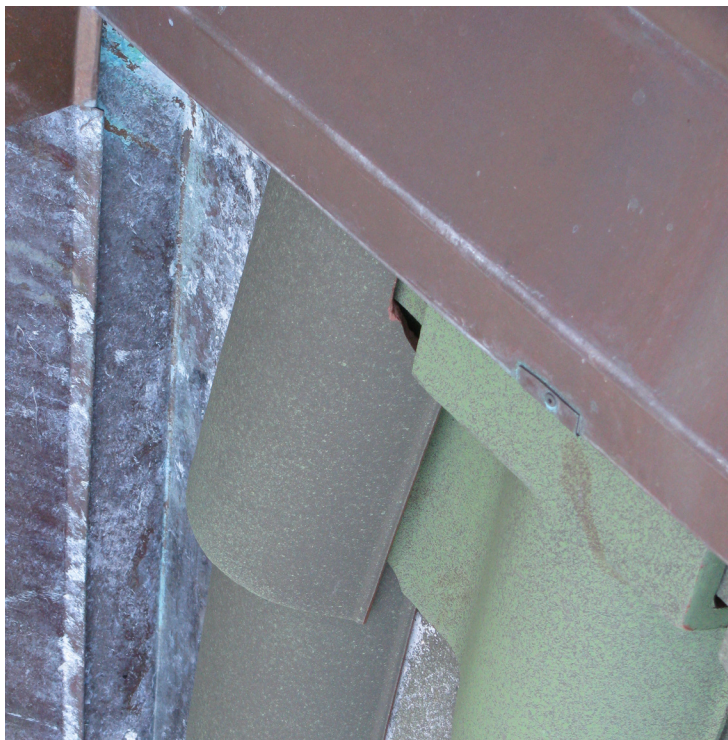
VS5: flat top tile not installed, tile loose and open to water
