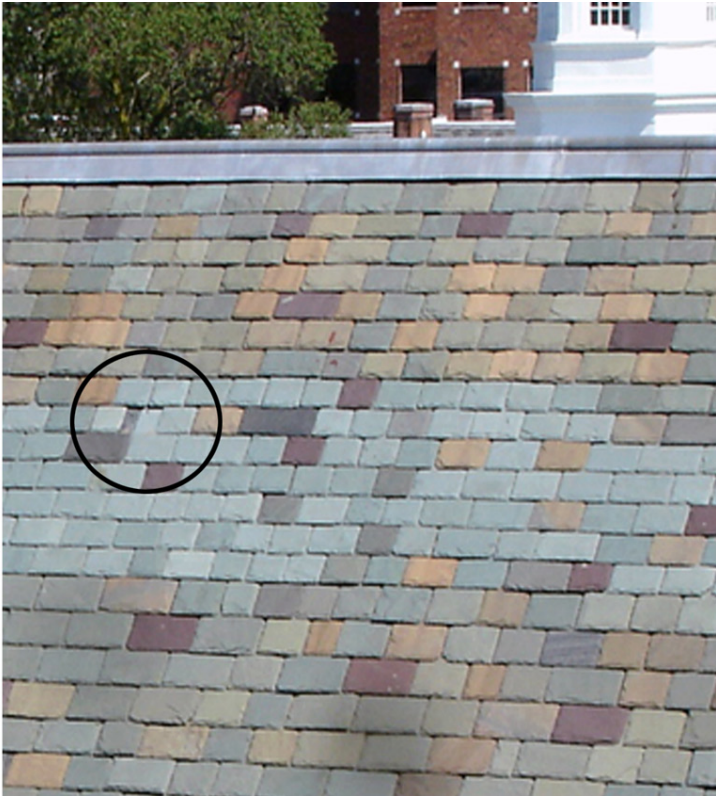
B6: slate missing four courses down from ridge and nine courses down from ridge
