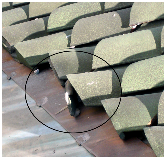
VS4: closed valley tile broken, past repair failed
