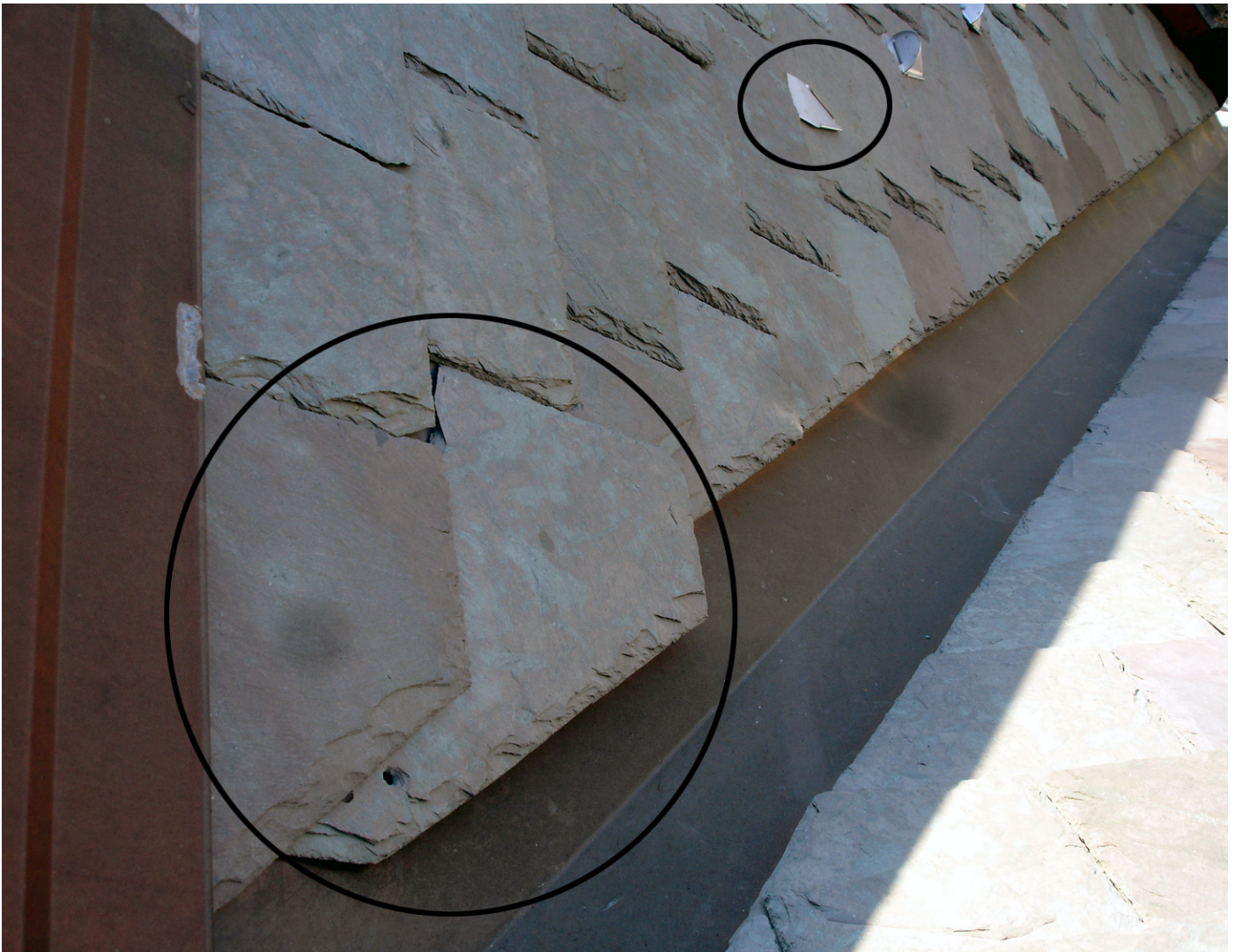
C2: slipping slate; smaller circle shows flattened snow guard
