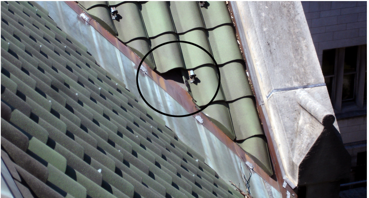
VS7: missing closed valley tile
